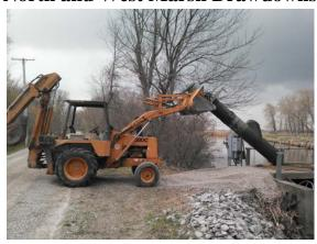
Removal of the broken lane pump
