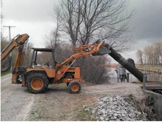
Removal of the broken lane pump
